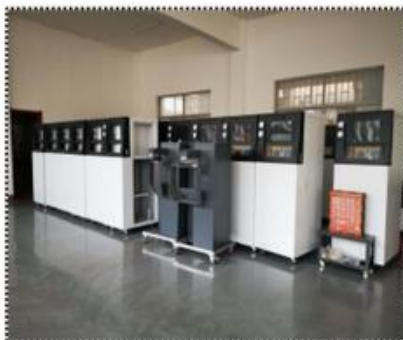
Control Cabinet Lab
